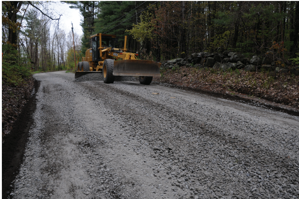
Center Road Reconstruction 2019
