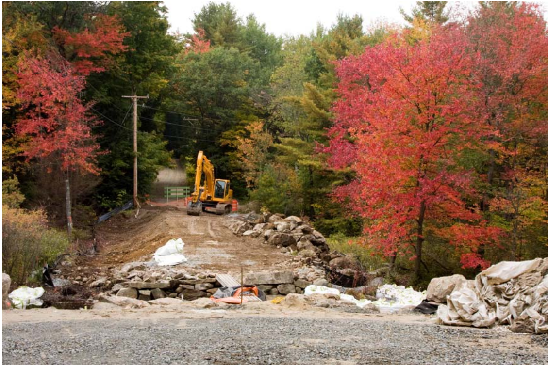
Gulf Road Bridge in progress by Nadine Preftakes
